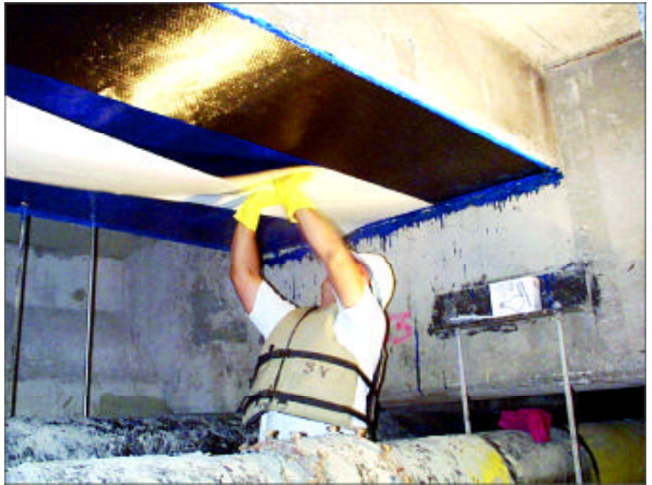
Figure 5. Applying Carbon Fiber Sheets to Underside of the Deck.
