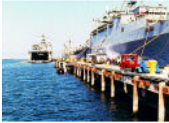
Figure 3. Pier 12 at San Diego.
