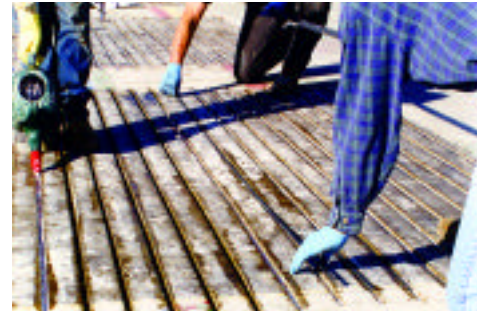
Figure 2. Placing Preformed Carbon Fiber Reinforced Polymer Rods Near the Top Surface.
