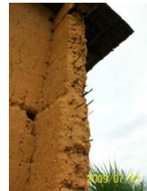
Fig.6: Exposed wall ribs
