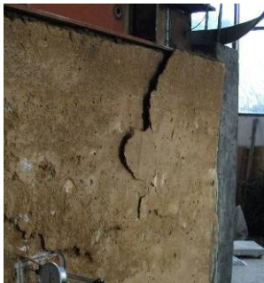
Fig. 5 Failure of W1
