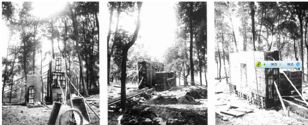
Fig.7 “Sculptor” construction site
