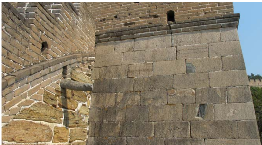
Quarried Stone. Water drainage spout. #8
