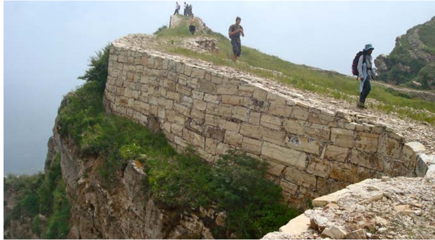
Figure 1. All stone, no brick, but Rubble Core. #13 and #14
