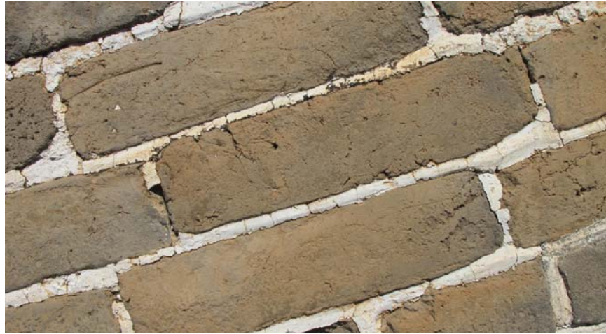
Figure 4. Sticky-Rice and Lime mortar. Typical brick. #5
