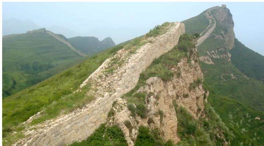
Figure 2. All stone, no brick, but Rubble Core. #13 and #14
