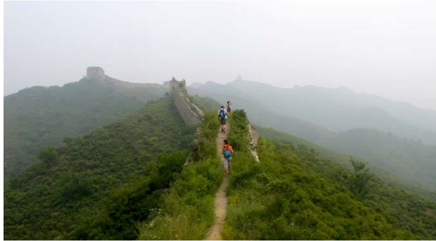
Figure 12. Outer walls brick walls slipped away. #5
