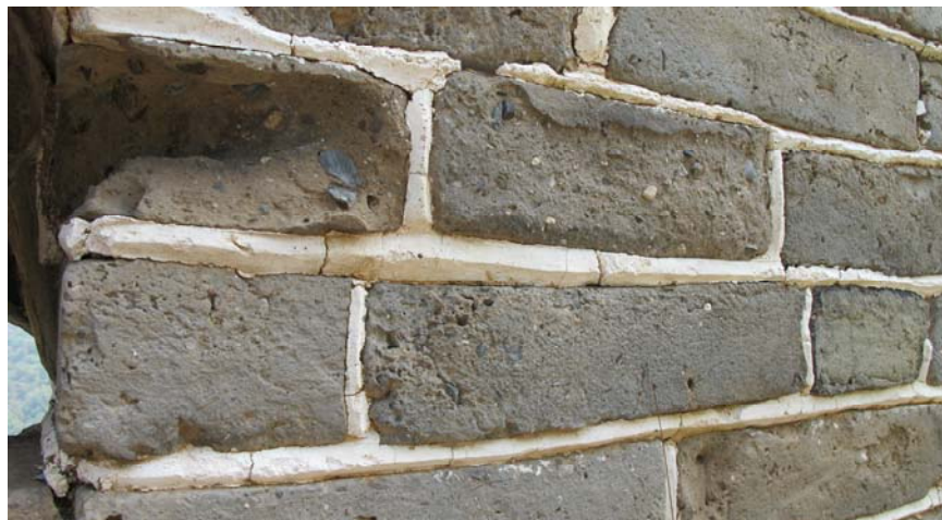
Sticky-Rice and Lime mortar. Typical brick. #8
