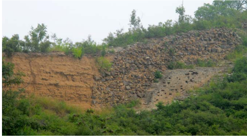
Figure 7. Rammed Earth and Rubble side by side. #5
