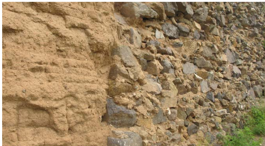
Rammed Earth and Rubble side by side. #5
