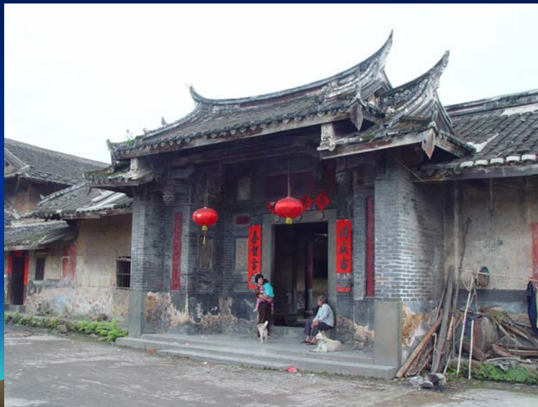
大夫第(永定) Da-Fu Building
