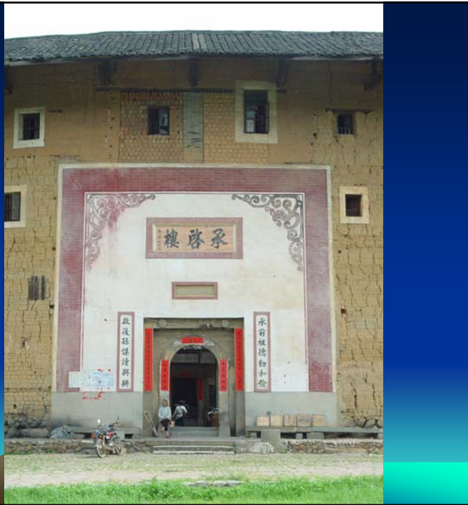
承启楼 Cheng-Qi Building
