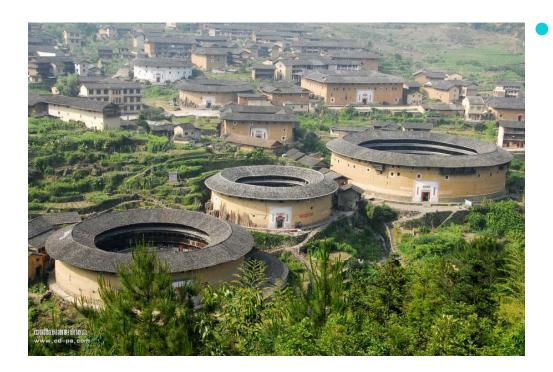
Hakka earth-buildings which are listed as world cultural heritages are located in Fujian- the coastal city where typhoons with heavy rainfall occur frequently. Its salient features are rammed earth wall and big picking eaves.
