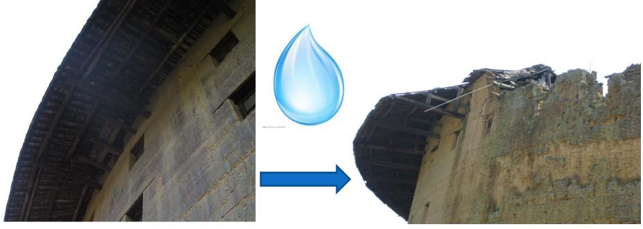
• In order to protect these important buildings, we should avoid all the negative factors. For rammed earth structures, as we all know, the biggest natural enemy is the rain. But for the Hakka earth buildings which have big picking eaves, wind driven rain is the greatest threat.
