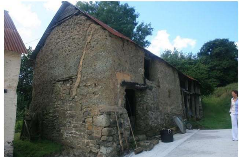
Cob barn adjacent to cob house. Devon, UK
