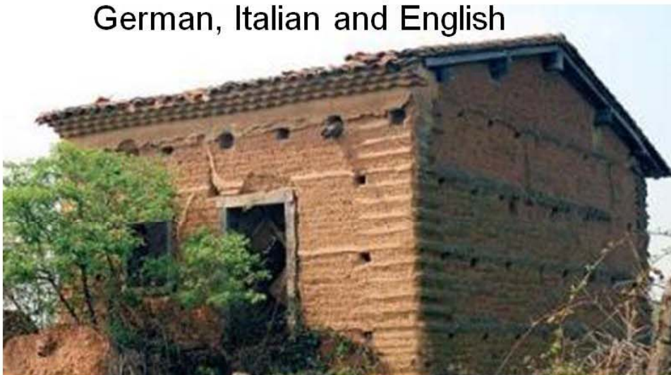
French rammed earth barn
