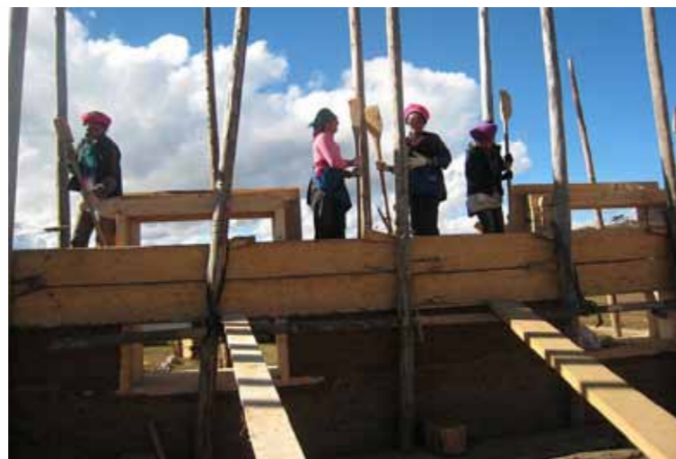
Rammed earth construction in Gyalthang (images: Yeshi Gyetsa)
