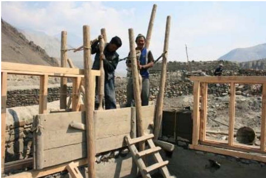
New rammed earth wall. Mustang region, Nepal
