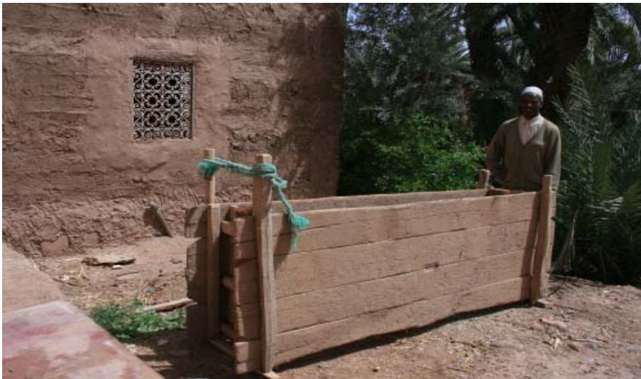
North African rammed earth formwork box. Asslim, Morocco.
