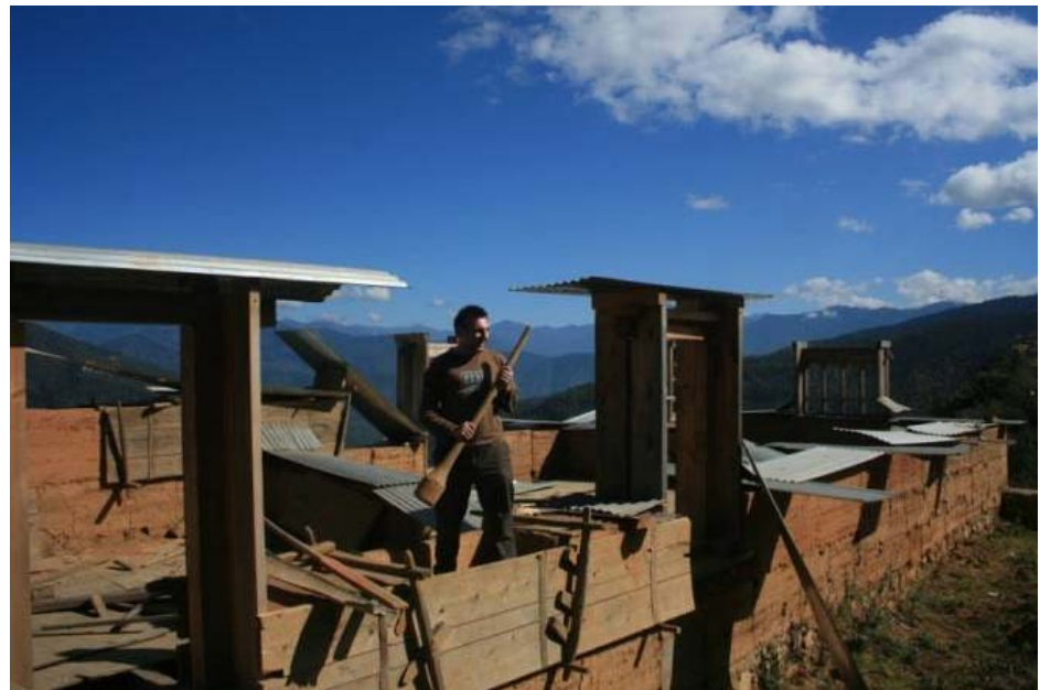
Part constructed rammed earth house in Bhutan
