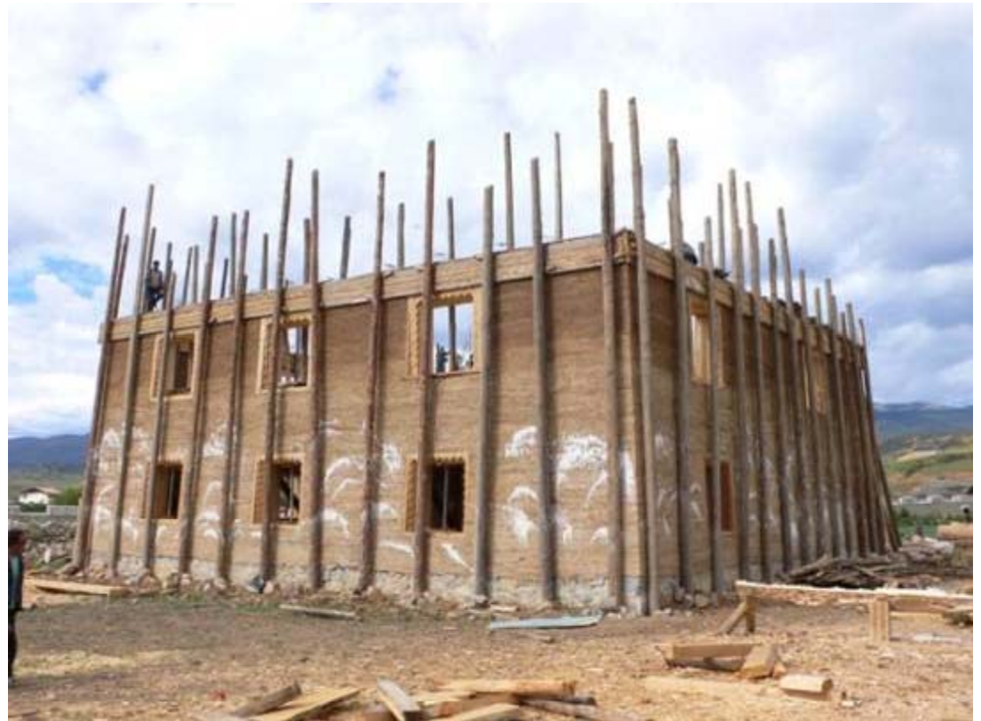
New rammed earth construction. Zhongdian County, Yunnan.
