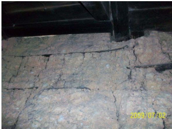
Rough rammed earth walls of Chengqi Tulou showing layer construction and wall ribs
