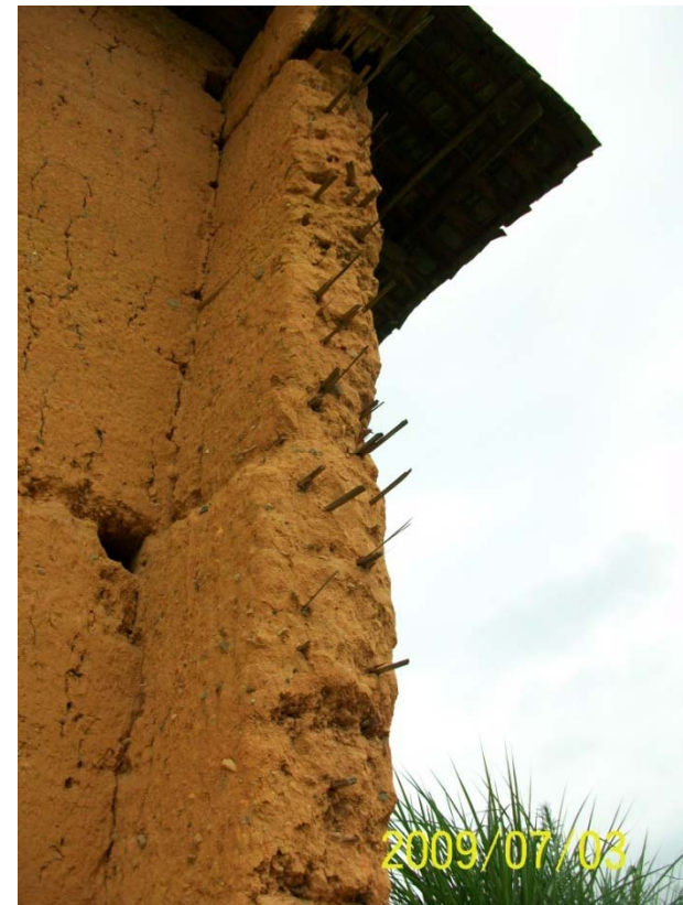
Pultruding wall ribs
