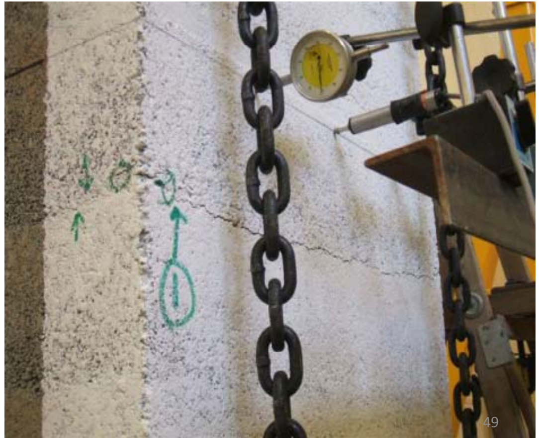
LVDTs and Cracks
