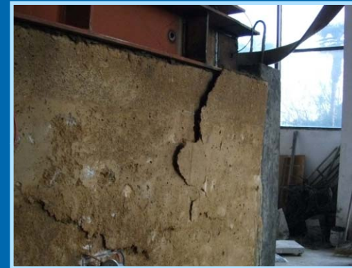
Crack grows rapidly
