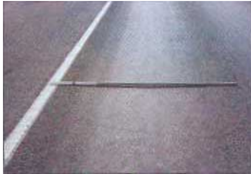
Figure D.7 Rutting
