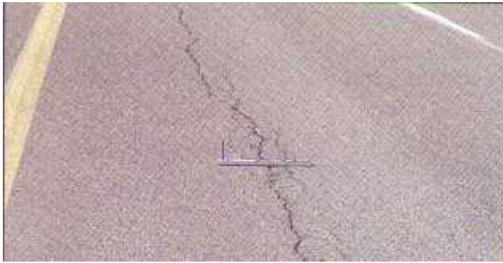
Figure D.3 Longitudinal Cracking
