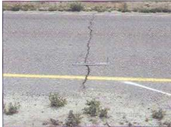
Figure D.4 Transverse Cracking
