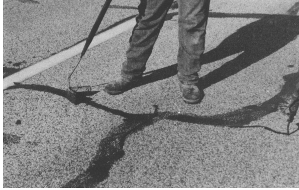
Figure 2.2 Crack Sealing
