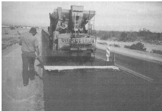
Figure 2.6 Slurry Sealing
